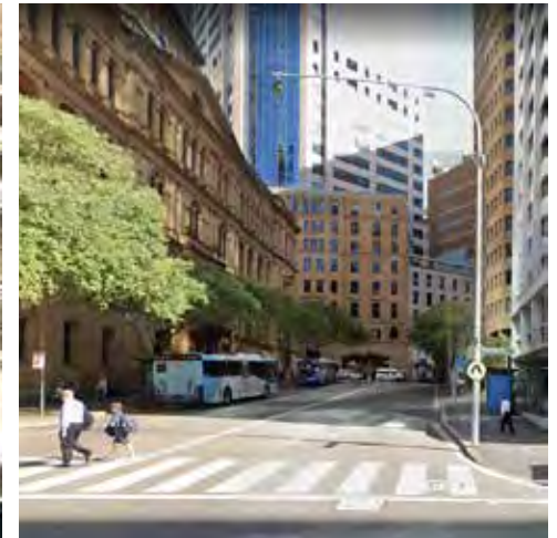
Gresham Street looking south at the Lands Department facade
